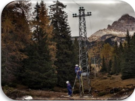
Overhead cables Structural level
