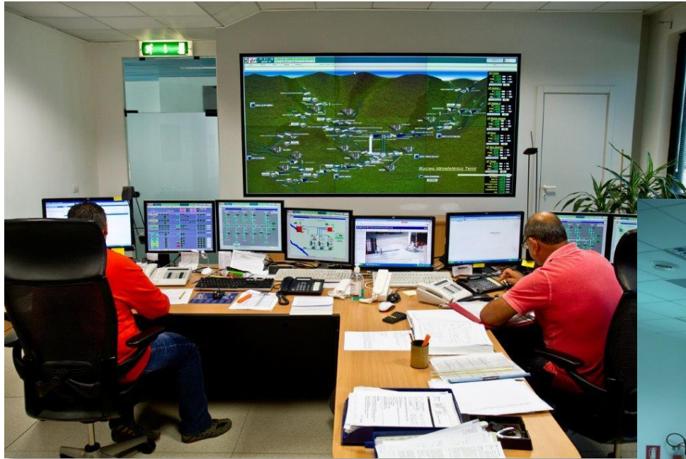
Control room with SCADA for thermo and bidding information (market access and trading through other systems)
