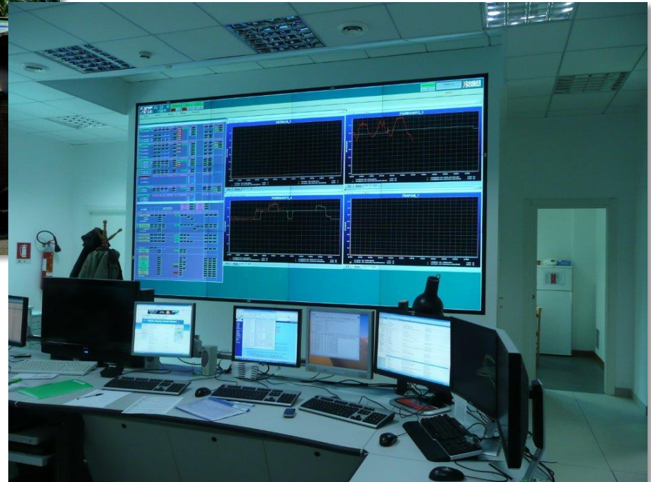
Control room with SCADA for thermo and bidding information (market access and trading through other systems)
