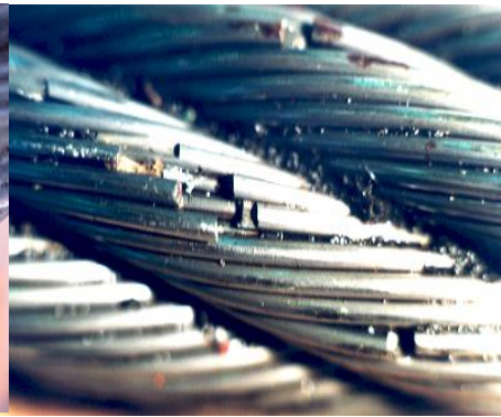
Fatigue broken wire
