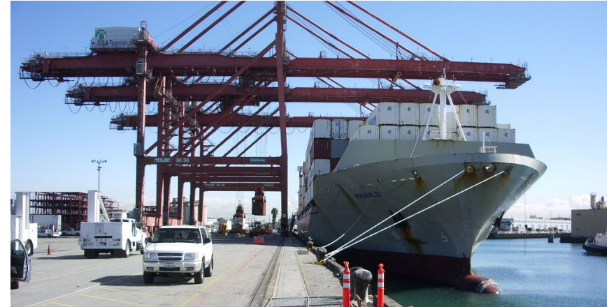
G. Parise, L. Parise, L. Martirano, P. B. Chavdarian, C. Su and A. Ferrante, "Wise Port and Business Energy Management: Port Facilities, Electrical Power Distribution," in IEEE Transactions on Industry Applications , vol. 52, no. 1, pp. 18-24, Jan.-Feb. 2016, doi: 10.1109/TIA.2015.2461176.
